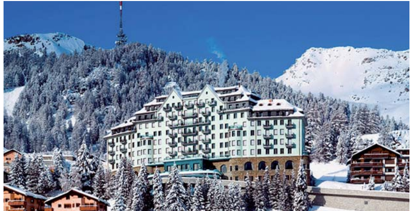
In the 5-star Ritz Carlton hotel in St Moritz, heat is recovered from waste water.
